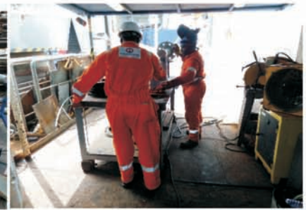
FINAL FABRICATION ON FLOW LINE AT UKPOKITI OFFSHORE
