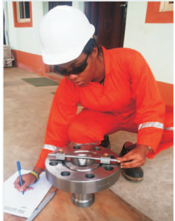
CHECKING BALL READING ON FLANGE
