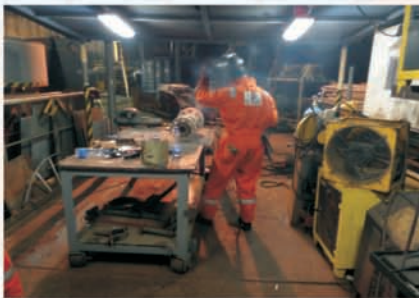
EVERPRAISE WELDER ON FLOW LINE PROJECT OFFSHORE
