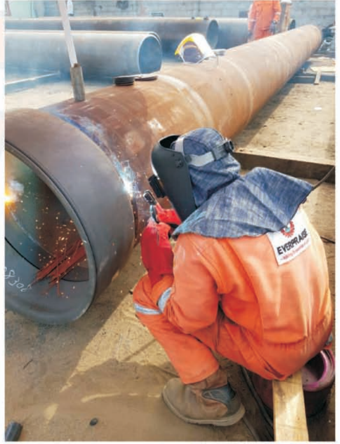
WELDING OF 30"X1" CONDUCTOR PIPES AND CONNECTORS
