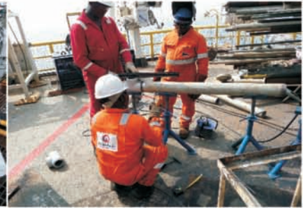
EVERPRAISE ENGINEER AND WELDERS, WELDING A TEE PIECE AT UKPOKITI OFFSHORE
