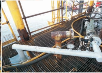
COMPLETE INSTALLATION OF FLOW LINE TO EXISTING HEADER
