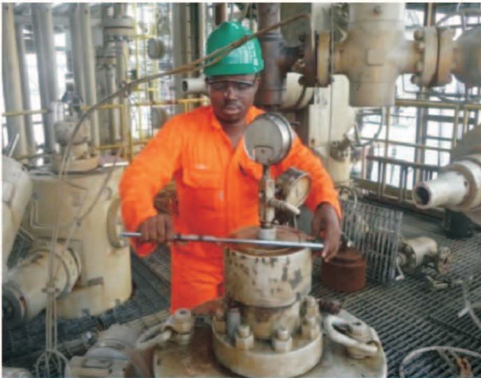
SITE INSPECTION OF WELLHEAD FOR MODIFICATION
