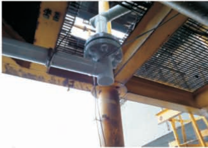
ANOTHER FLOW LINE INSTALLED BY EVERPRAISE
