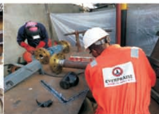
PRE-FABRICATION OF FLOW LINE IN EVERPRAISE BASE AT UKPOKITI OFFSHORE
