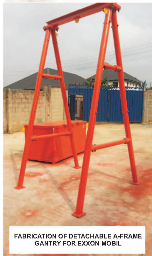
ON-GOING FABRICATION OF DETACHABLE GANTRY
