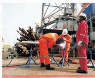
WELDING OF FLOW LINE AT UKPOKITI OFFSHORE
